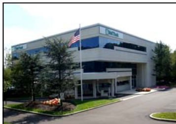
3 STORY CLASS A OFFICE BUILDING
