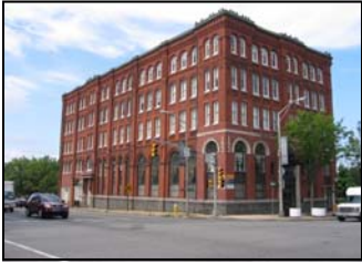
MULTI-STORY BRICK OFFICE BUILDING
